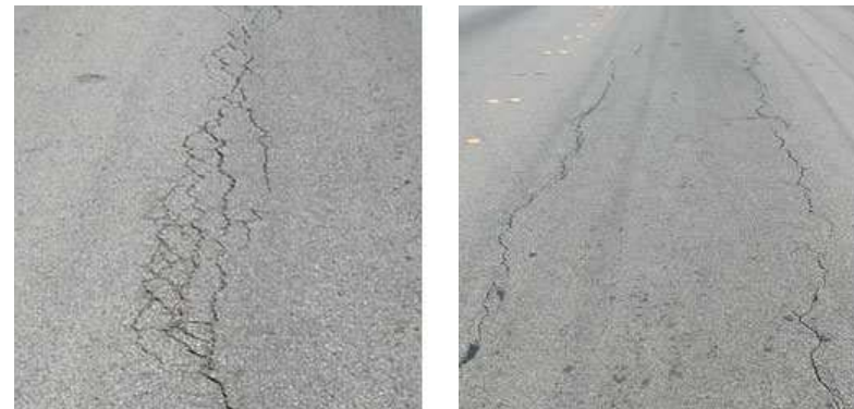
Fatigue cracking
