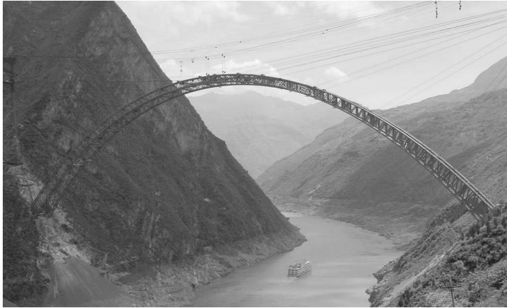
Figure 5: The view of arch rib tube truss closure of Wuxia Yangtze river bridge
